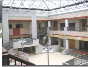
Guilford County Schools Northern Middle School and Northern High School
